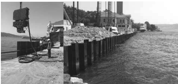
Figures 12a and 12b Sheet Piling
