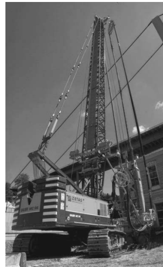
Figure 8. Diaphragm Wall Machine, Hydrofraise-Cutter
