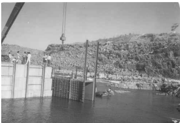
4.10 Masonry Works above water level.
