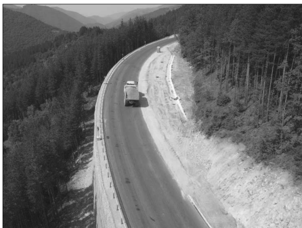
Figure 9. Top view of a completed GRS-wall.
