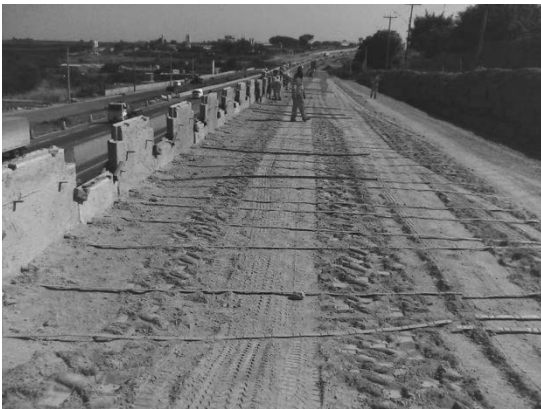
Figure 5. General view of the top part of the reinforced soil fill.
