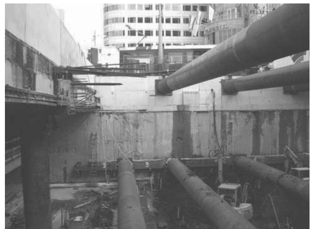
Figure 1. Building pit of car park Kruisplein.
