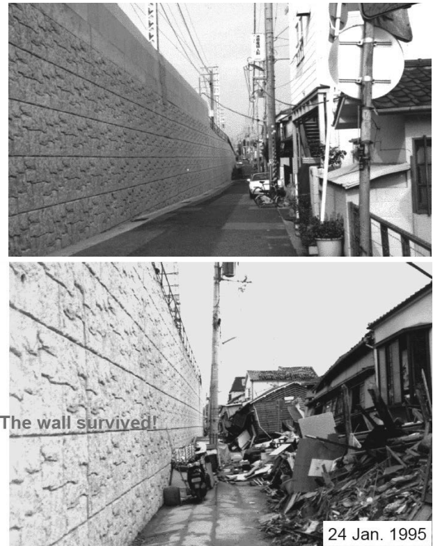
Figure 3. Geosynthetic reinforced soil structure (GRS structure) as railway embankment after completion 1992 and after the Kobe earthquake 1995 (Tatsuoka 2008).
