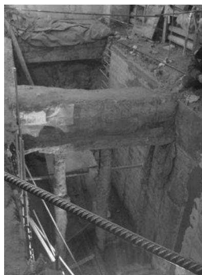
Figure 8. 4.5 m deep service duct
