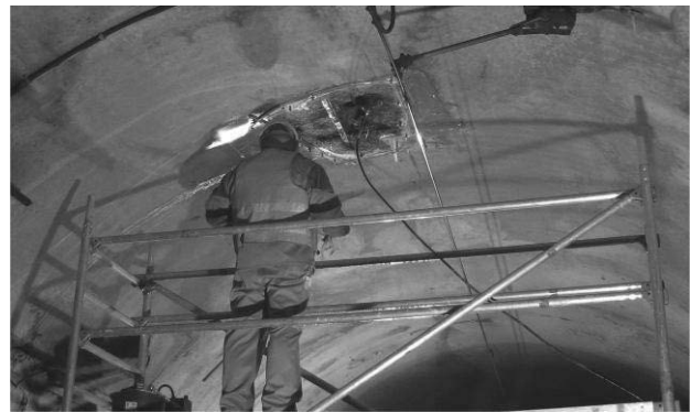
Figure 4. Main inspection in a tunnel.
