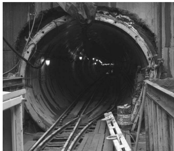
Figure 2. Service tunnel construction on Gruzinsky Val Str. In Moscow.
