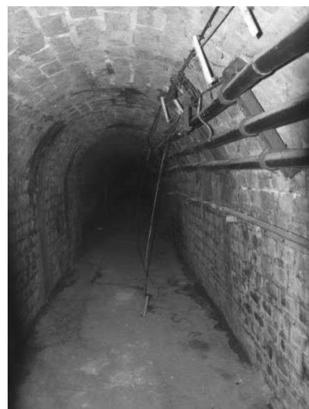
Figure 2. The tunnel with the concrete masonry support system
