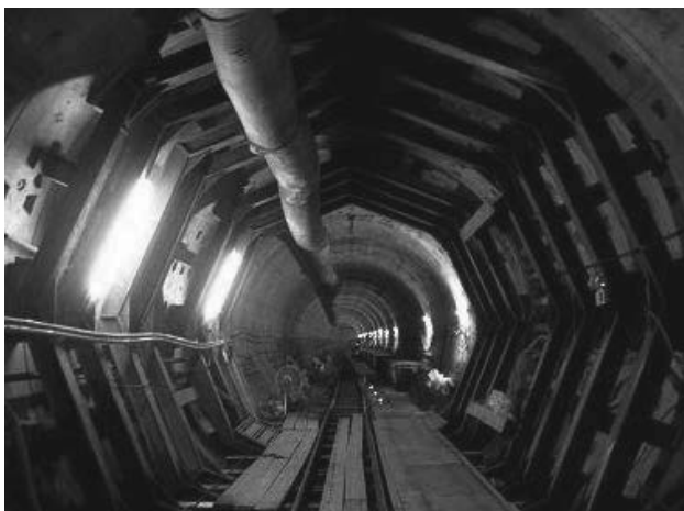
Figure 9. Octagonal steel-beam reinforcement inside tunnel.
