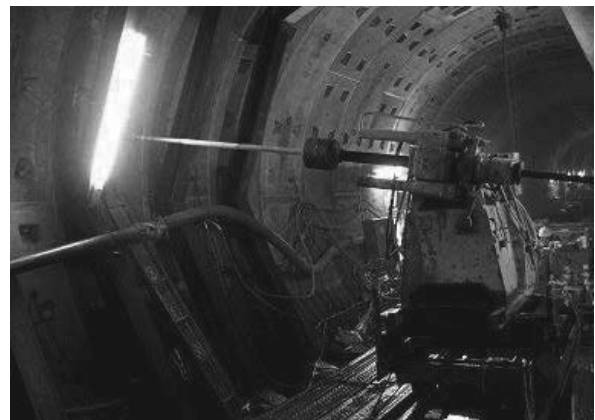
Figure 7. Additional chemical grouting in tunnel before cross passage excavation.
