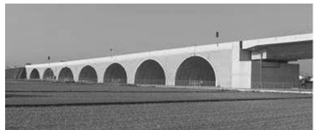
Figure 1. Multi-arch culverts embankment
