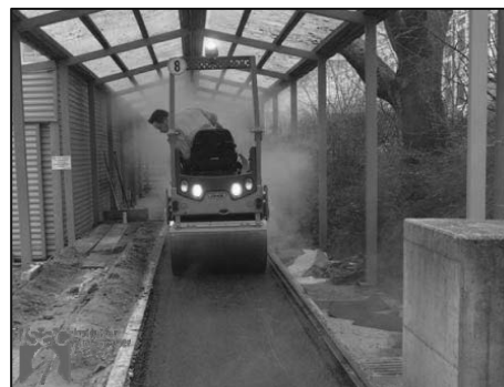
Figure 4: Wearing course compaction
