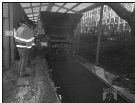
Figure 3: Wearing course installation
