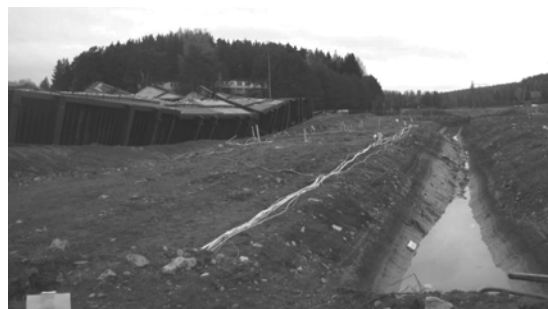
Figure 1 Test site after the failure. Instrumented area is between the containers and the ditch. Loading structure has overturned and the slip surface is protruding from the ditch.
