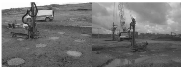
Figure 7. Execution of the Ménard pressuremeter between and centrally in the columns
