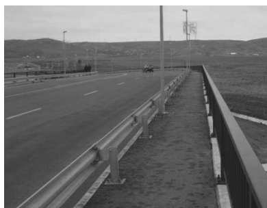
Figure 3 Longitudinal view of the embankment.
