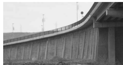
Figure 2 Lateral view of the embankment.
