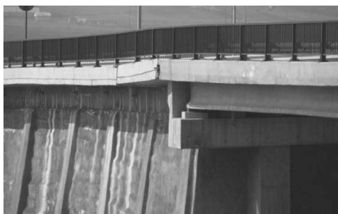
Figure 4 Zone between embankment - bridge.
